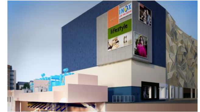
Underground 132 kV SS at 'Quest Mall'
